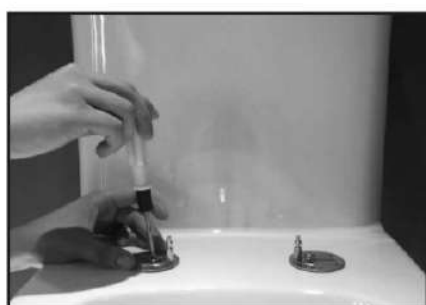
4. Once positioned correctly, tighten the screw fully and fit fixing cover
